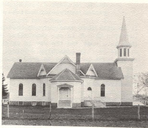
The rebuilt St. Pauls Church of 1902
